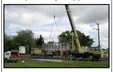
truck and unload on site placing the top onto the base which was then secured to the platform using trubolts.
