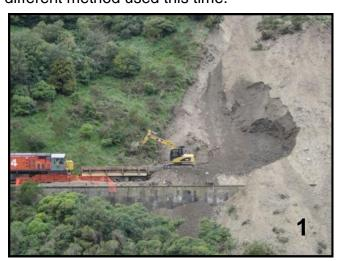
The first picture shows the way it used to be done. An excavator has been unloaded and the work train consisting of one wagon and a diesel locomotive is positioned to allow the excavator to load the wagon. When loaded the wagon will be towed away to where it can be unloaded, before being returned for the excavator to load again.
