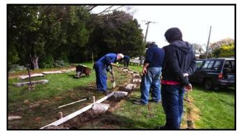
The rails were scrubbed with a rotary wire brush and then painted with 'cold galvanising' paint.
