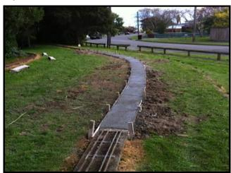
The following Thursday the boxing was removed and dirt was reinstated next to the concrete. The club's ride on mower was used to compact the dirt. The painting of the rails was completed and new holes in the sleepers were drilled ready for the 'Dyna-Bolts' which hold the rail down to the concrete. Off site strips of conveyor belting were cut ready to glue on to the sleepers before the rail is re-laid.
