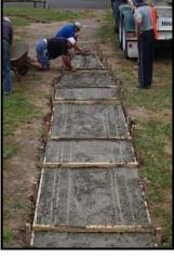
The section incorporating the Y turnout and two parallel roads was then boxed up and the prefabricated tracks and turnout were suspended and positioned on the formwork with concrete poured the next day.
