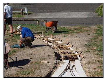
The curved track section was next boxed up and the track fabricated and welded up insitu suspended on the formwork, concrete again
